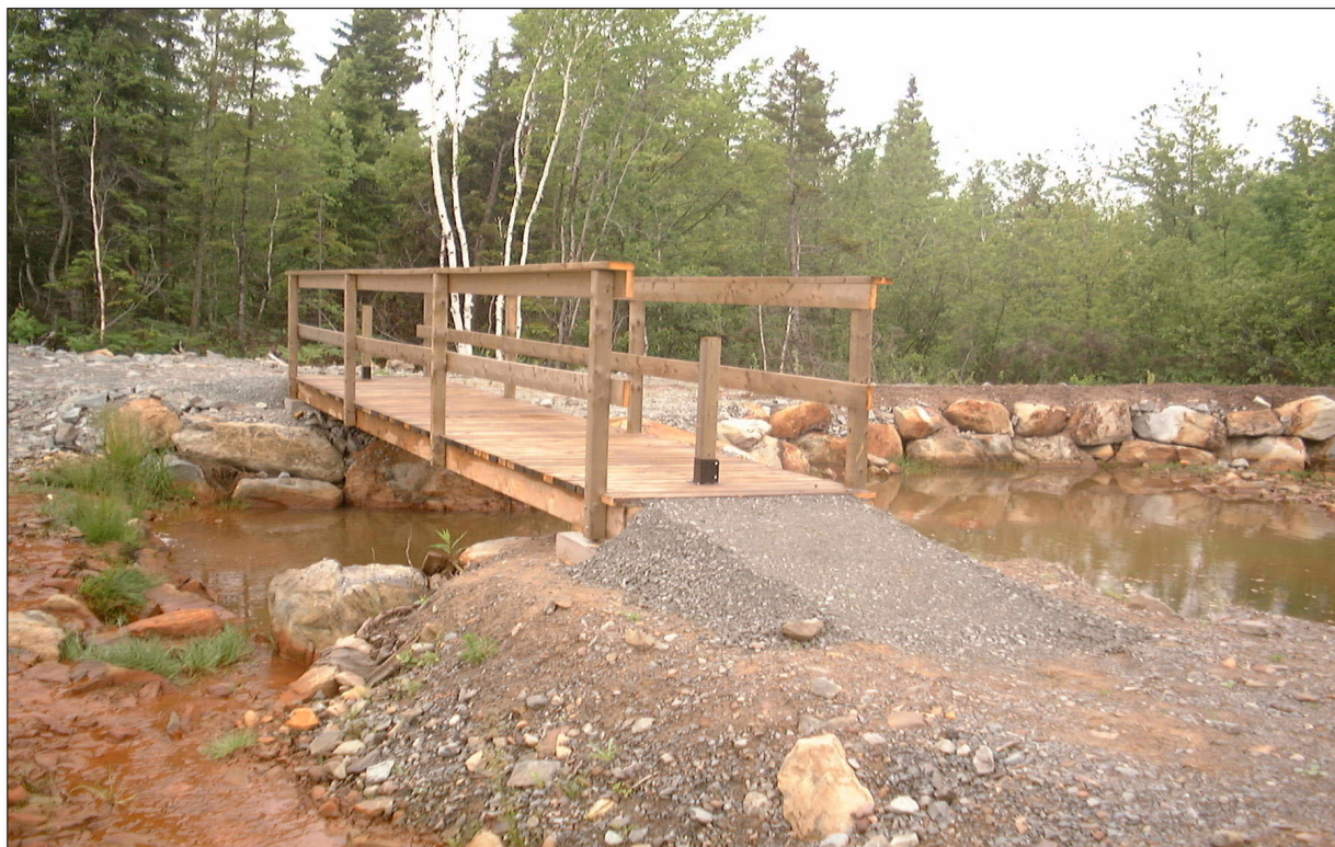
Figure 12. One of the wooden bridges.
