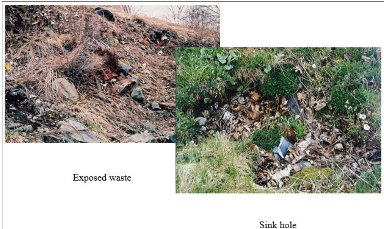
Figure 5. Exposed waste and sink holes in former landfill (current sport field).
