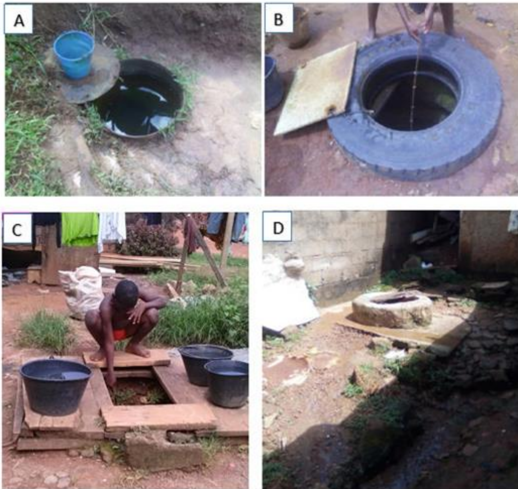
Figure 3. Examples of the most common groundwater extraction devices and structures in the Melen Slum: (A) limited protection well; (B) Protected well with lid in poor condition (limited protection); (C) Unprotected well; (D) Protected well with no lid (limited protection).
